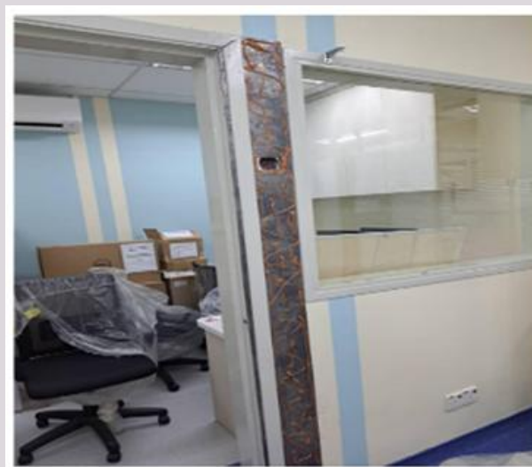
Figure 1: Lead sheet installed to a door frame of an X-ray room
