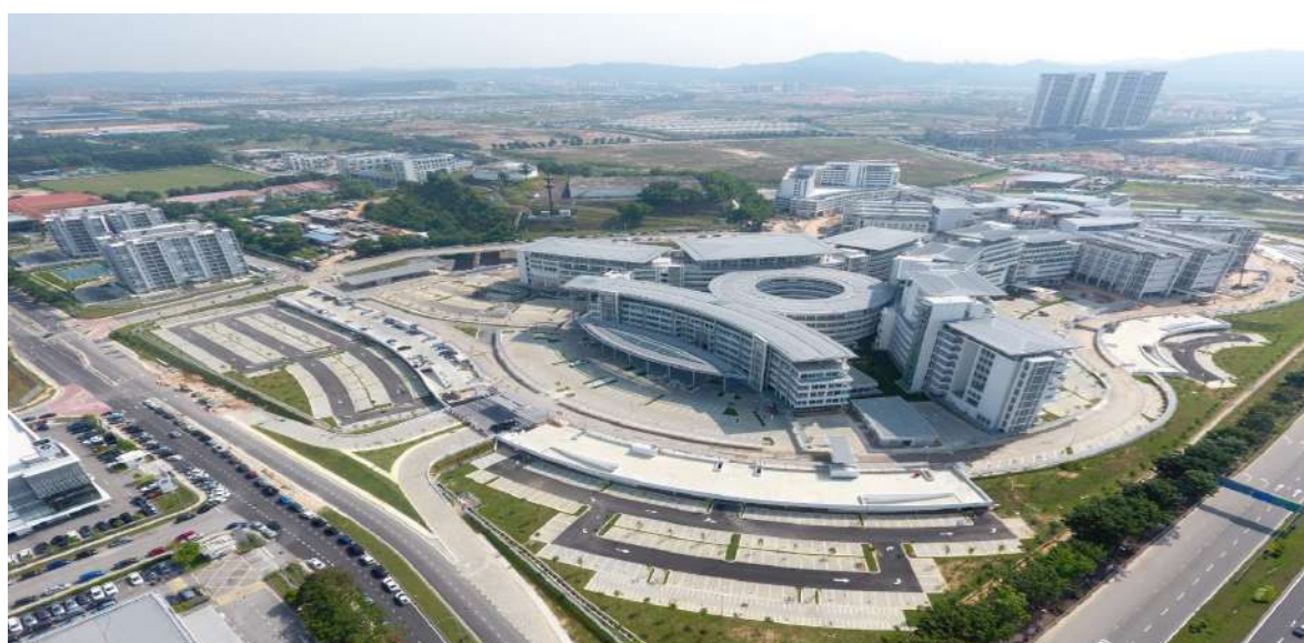
Image 17 NIH New Complex
