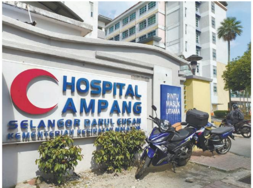
Dzulkefly said the Health Ministry has directed a comprehensive structural and digital audit of Hospital Ampang to address underlying issues stemming from its ageing infrastructure. — ADIB RAWI YAHYA/THESUN
