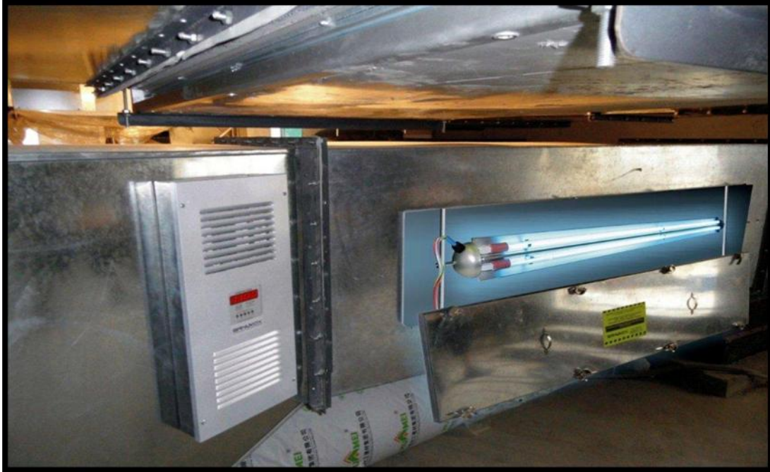
Figure 1: UV Bio-Wall In-Duct Air Purifier creates a "barrier wall" of UV energy which destroying biological and chemical contaminants. It is mounted parallel to the airstream in order to maximize the contaminant's contact time with the UV energy. (courtesy from [REDACTED] Technologies Inc.)
